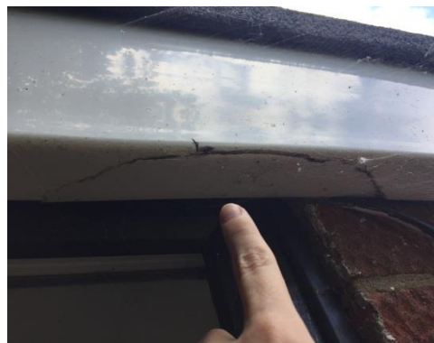
Large crack to the doorframe
