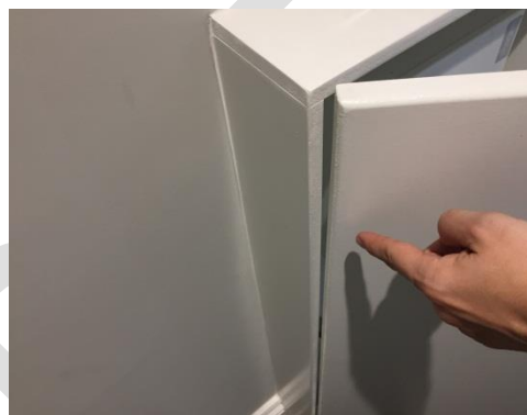
Cupboard door loose to the hinge
