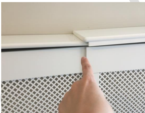
Radiator housing screw loose, leaning inwards
