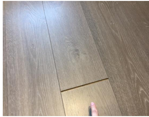
Gapping to floorboards
