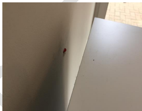
Radiator housing loose to wall
