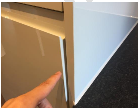
Freezer unit door loose to top hinge
