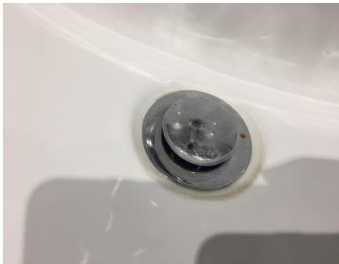
Sink pop up not working/ scaled waste
