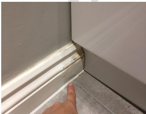
Water damage to skirting
