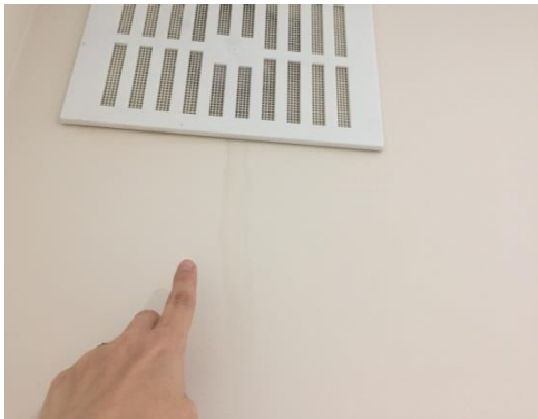
Water staining under the vent
