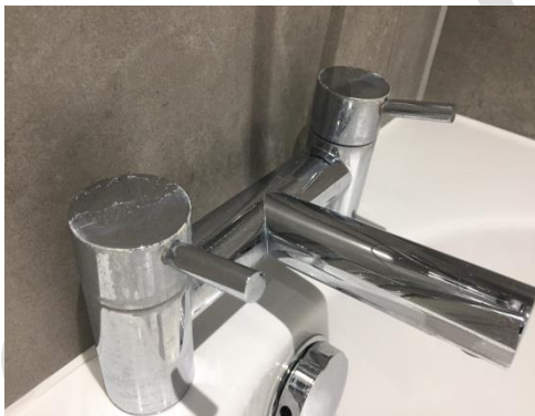
Scaled bath mixing controls
