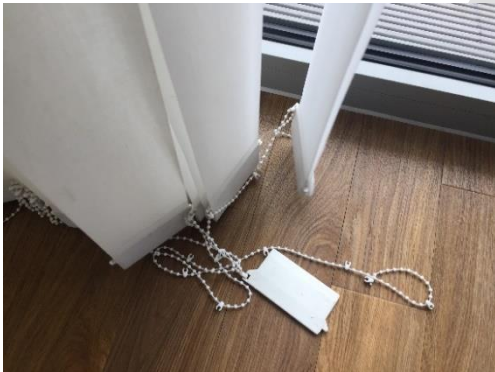
Blind slats detached from the base cable
