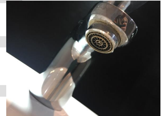
Scale residue on the sink tap spout
